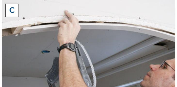
different sized openings, I like to use segmented arches, since the arches can be made with the same spring line and rise. Elliptical arches can also have the same spring line, rise, and finished opening height, but some types of corner bead are difficult to bend along the tightly radiused areas of the arch.
